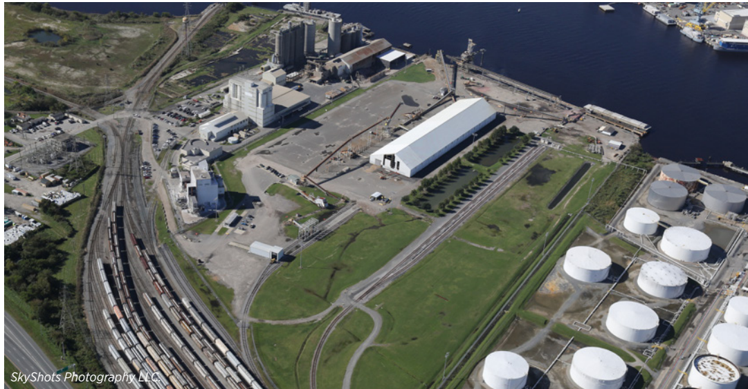
In Virginia, VHB is performing land surveying and planning, engineering, and permitting for the redevelopment of land in several key ports, including Seagate Marine Terminal (bottom right) and Kerneos site (top left) in Chesapeake.
